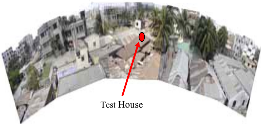
Figure 2: Physical condition of Test house area (Gulshan) in Dhaka city
