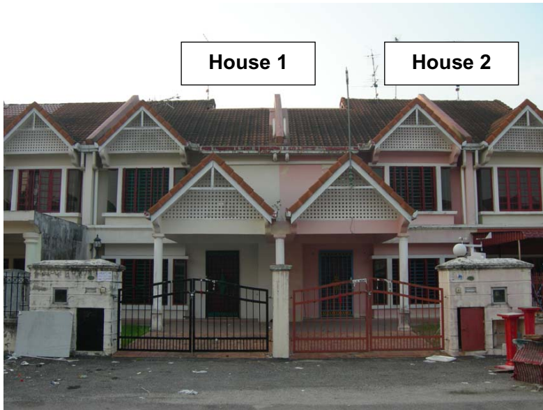
Figure 2. Front view of the case study houses.
